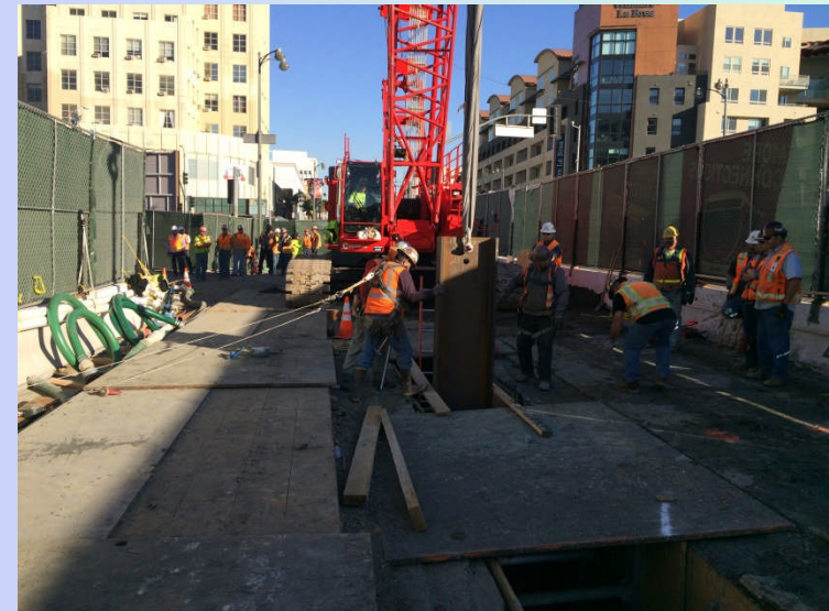
Installation of the first Wilshire/La Brea Station Pile
