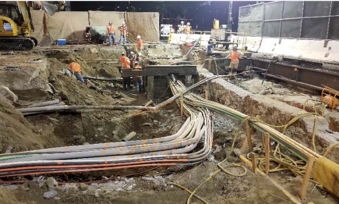
Utility work on Flower Street
