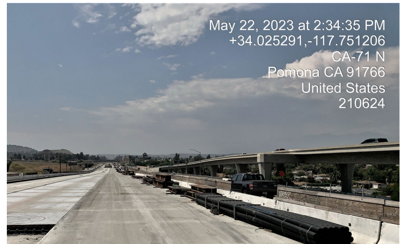
JPCP paving in the median
