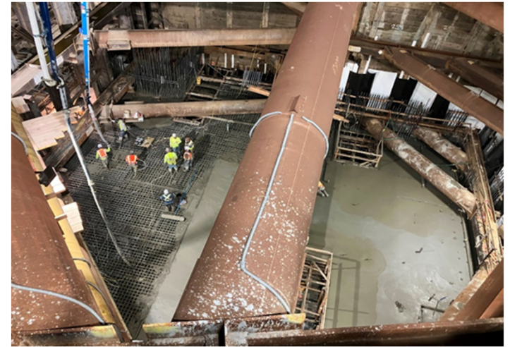
Westwood/UCLA Station: Concrete Placement for Main Entrance Invert
