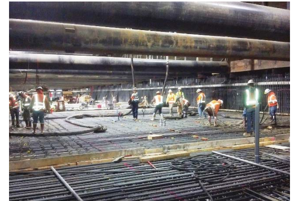
Wilshire/La Brea Station
