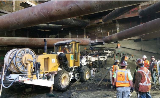
Drilling and Installing Canopy Pipes for SEM Cavern at Broadway Station
