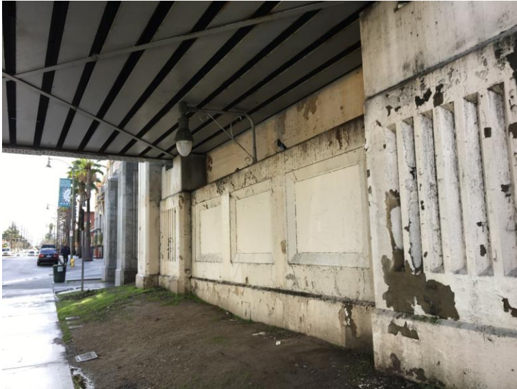
Lincoln/Cypress Station - Before
