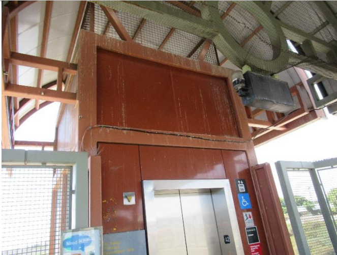
Vermont/Athens Station - Before
