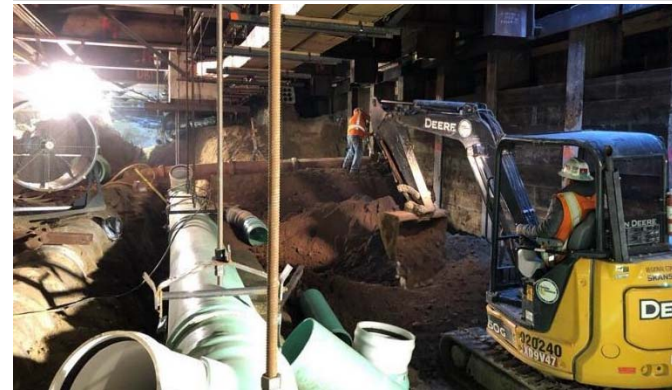
Preparations for sewer bypass under Flower Street
