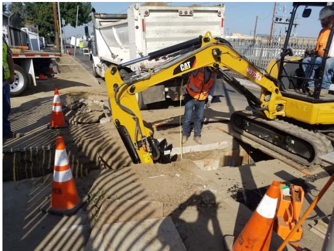
UG conduits crossing the street
