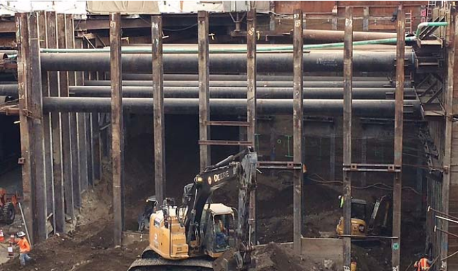
Excavation at Alameda Wye
