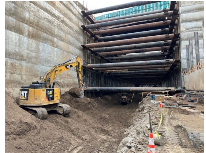
Westwood/VA Hospital Station: Excavation in Station Box
