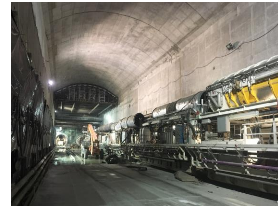
TBM Gantries at Wilshire/La Cienega Station
