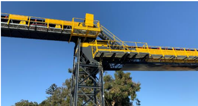
Conveyor Belt Assembly for TBM Operation at Tail Track Exit Shaft
