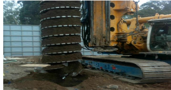
Drilling for Support of Excavation Soldier Pile Installation at Westwood/VA Station
