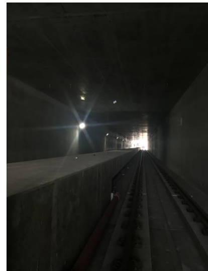
Center walkway at UG-1 Area for lighted handrail, 4-inch wide thermoplastic edge striping, overhead lighting adjustments, power circuits, and redundant circuits
