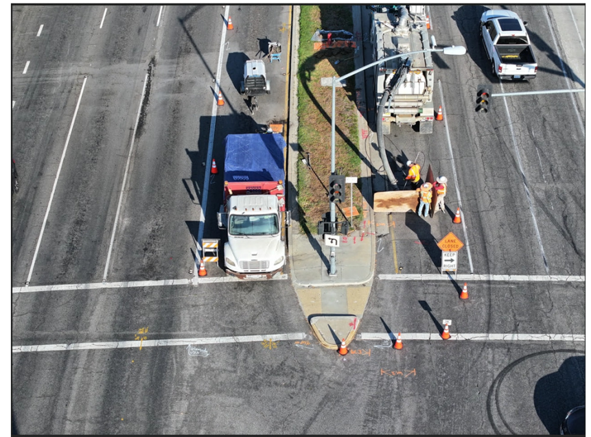
Potholing in Glendale
