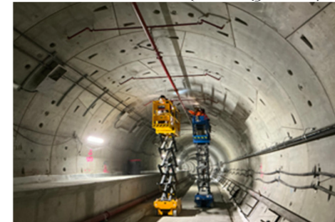
Tunnels: Tunnel Lighting Installation Reach 7 BR Tunnel
