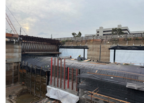
Westwood/VA Hospital Station: Roof Rebar Installation (Looking South)
