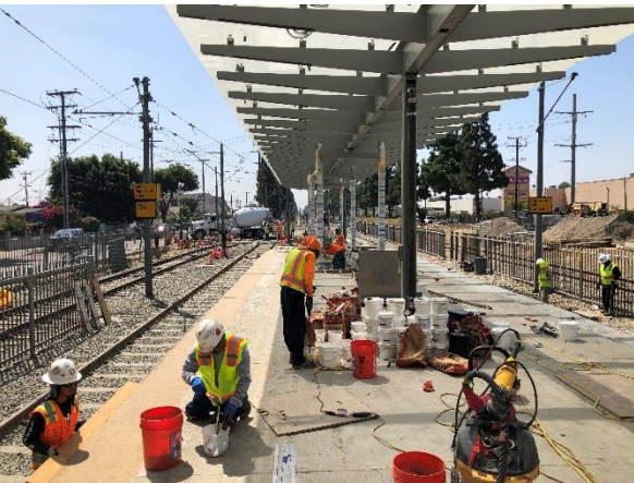
Blue Line Platform Work
