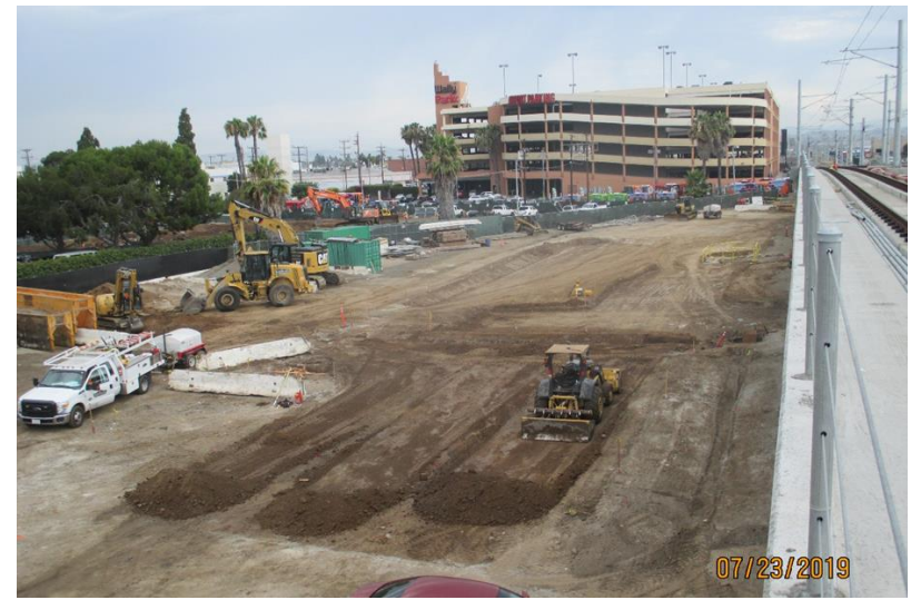
Grading for Aviation/Century Station plaza and parking lot
