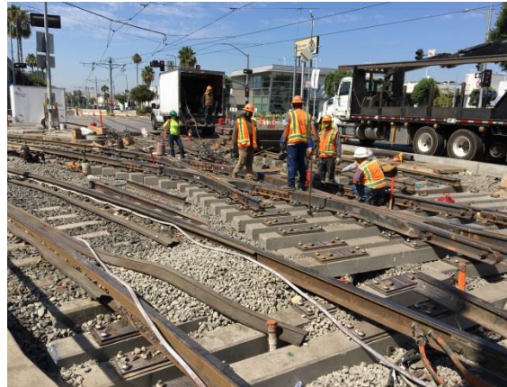
Replacing trackwork at Expo Junction
