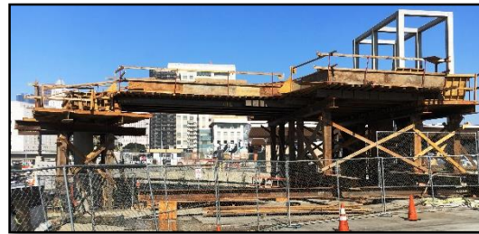
Elevator Platform Falsework
