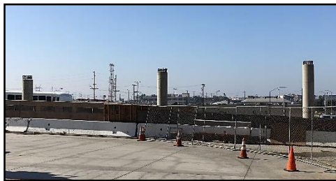
Pedestrian Walkway Columns
