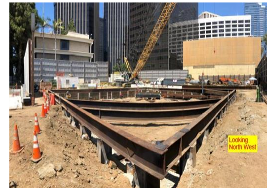
Tunnel Shaft Excavation in Century City
