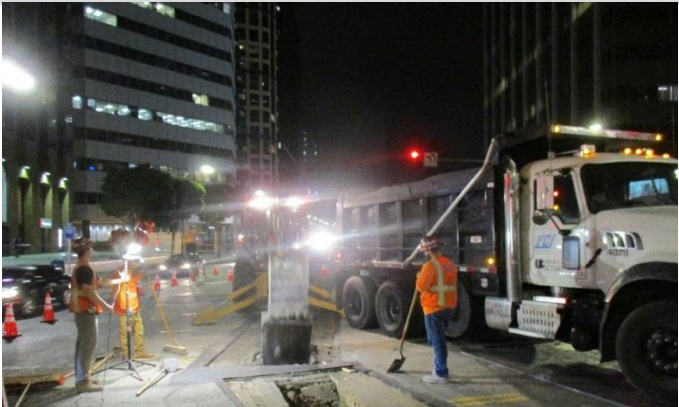
Main Line A Excavation and Potholing
