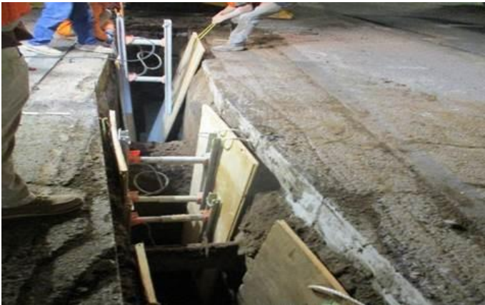
Hand Dug Excavation for Fiber Optic Conduit
