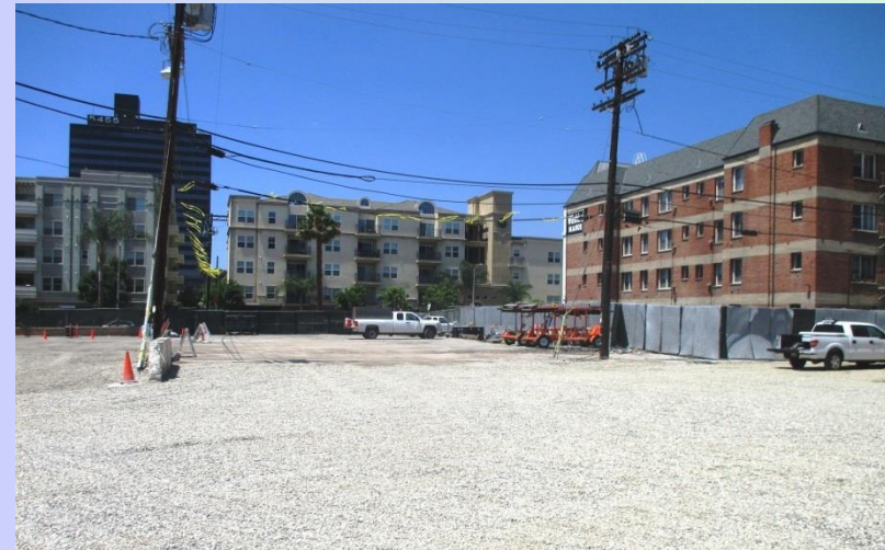
Site Preparation at Wilshire/La Brea North Yard
