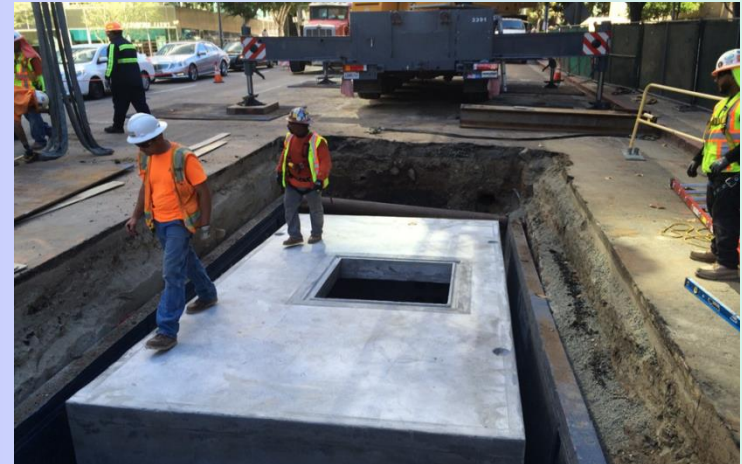
Vault installation on 5 th /Flower intersection
