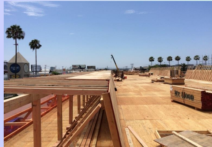
AVIATION/CENTURY STATION – Bridge falsework for concrete pour
