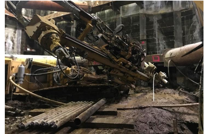
Westwood/UCLA Station: Soil Nail Operation at the West End Wall
