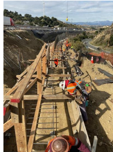
Rebar Installation at Retaining Wall 2460
