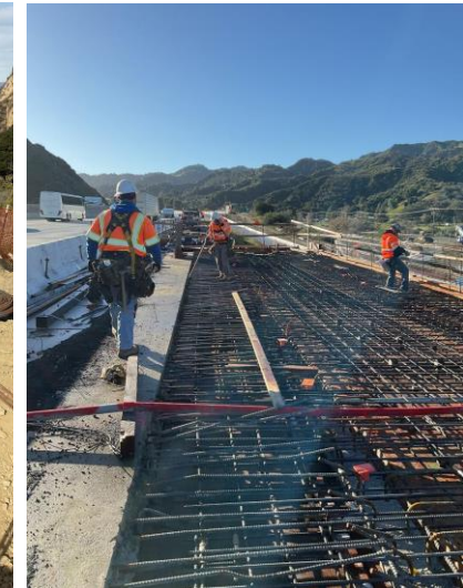
Preparation for concrete Pour of deck at Calgrove Blvd.
