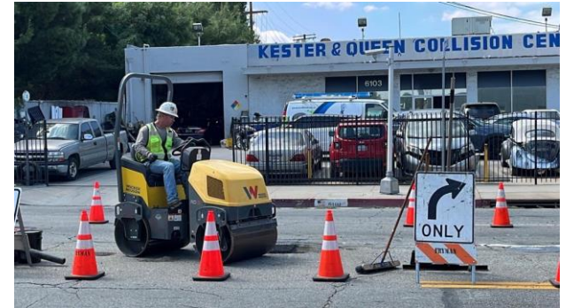
Potholing Restoration on Bessemer St.
