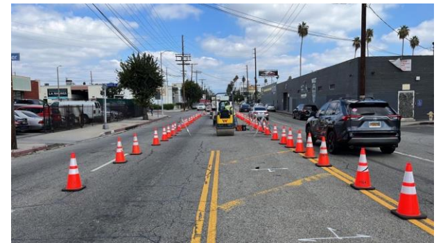
Pothole Restoration on Kester Ave
