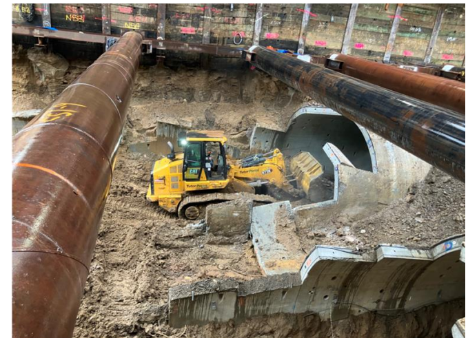
Westwood/VA Hospital Station: BR Tunnel Liner Removal in Excavated Station Box
