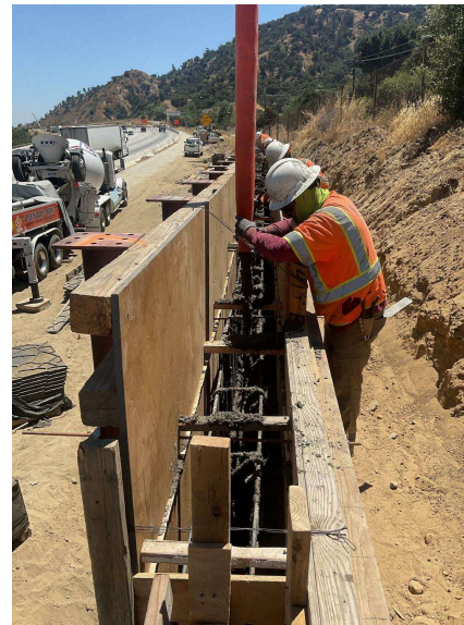
Pouring concrete at Retaining Wall 2461
