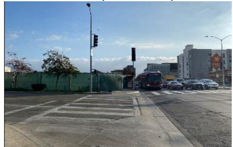
Intersection of Van Nuys Blvd. & Keswick St.
