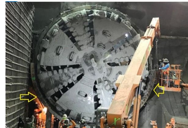
Purple TBM Arrival of Wilshire/La Cienega Station
