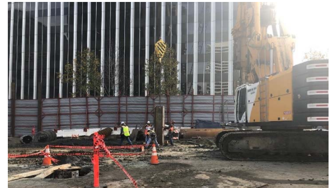
Soldier Pile Installation in Century City
