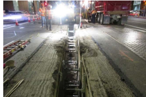
Ductbank Trench Excavation
