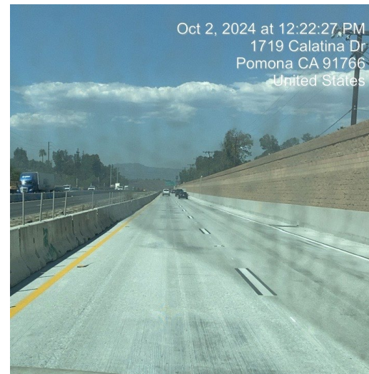
NB-71, completed stage 1 roadway.
