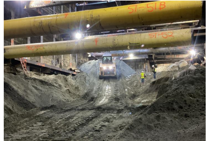
Century City Constellation Station - Excavation Progress
