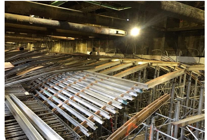
Wilshire/Rodeo Station - Station Box Roof Deck Form Work
