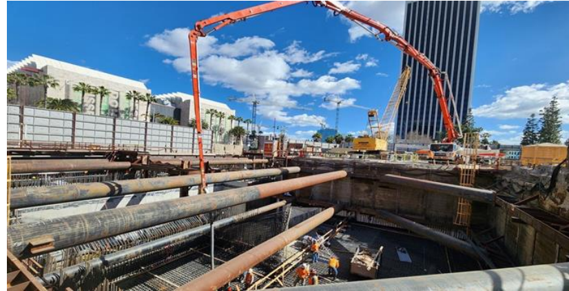
Wilshire/Fairfax Entrance Structure Deck Placement
