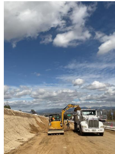
Structural Excavation for RW-2708
