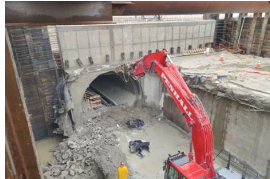
West Portal Wall Demolition
