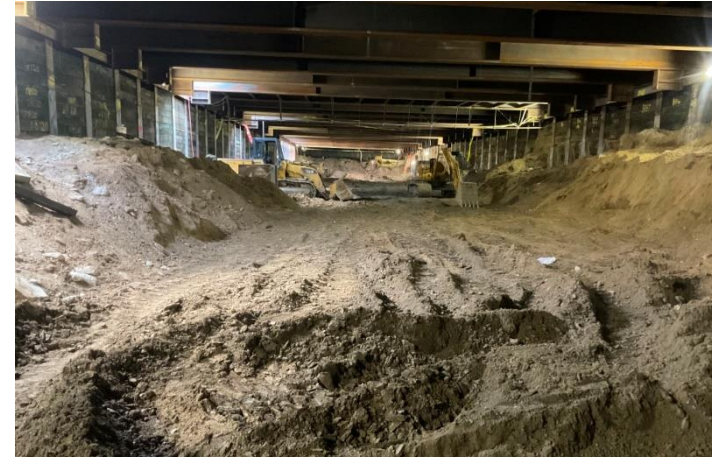
Westwood/UCLA Station: Excavation underneath Wilshire Blvd
