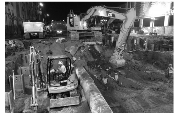
Contractor exposing utilities on Wilshire Blvd. & Orange Drive
