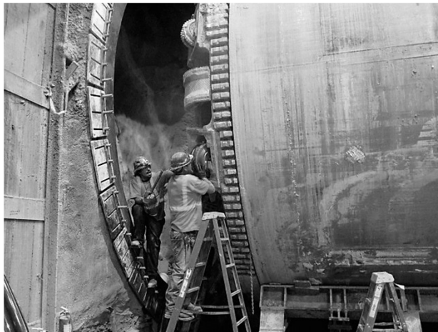
TBM ready for relaunch to Leimert Park Station Box
