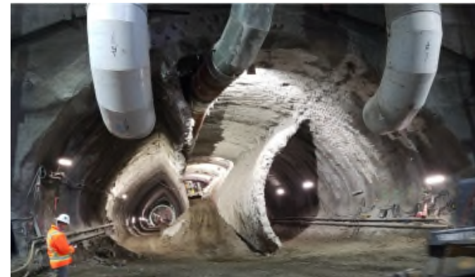
Demolition progress of central walls of SEM
