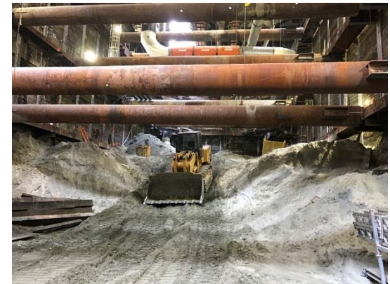
TBM Launch Box Excavation in Century City
