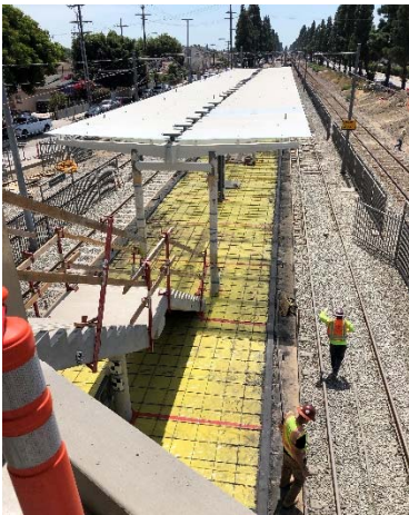
Blue Line Platform Work
