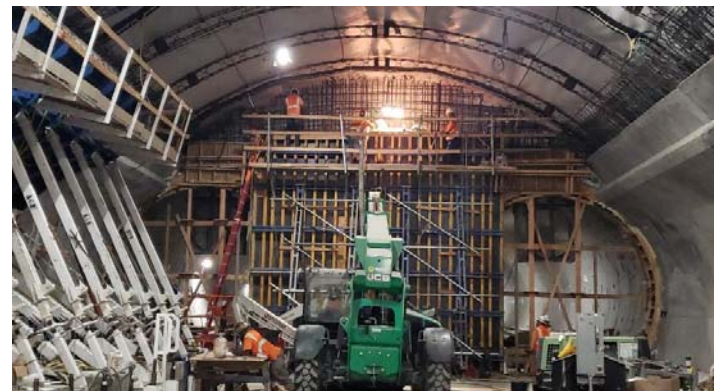
Concrete placement of headwall in SEM Cavern
