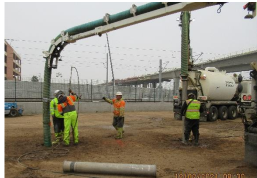
Potholing for Stormwater Capture System
