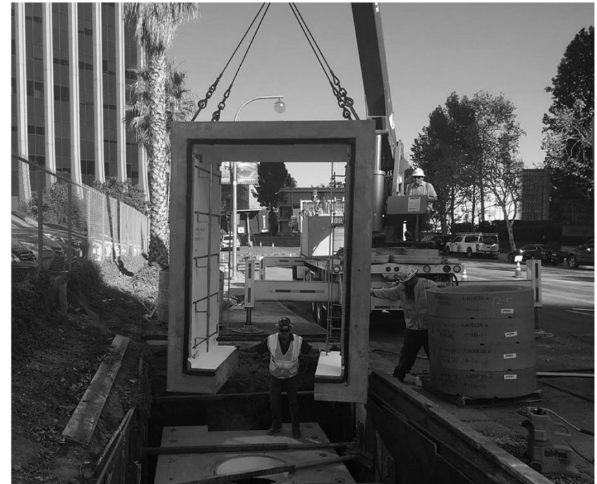
AT&T CA manhole Installation in Century City
