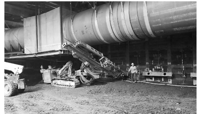
Tieback installation at Historic Broadway Station
