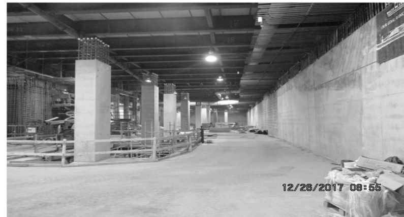
Concourse level columns and walls at Leimert Park Station
