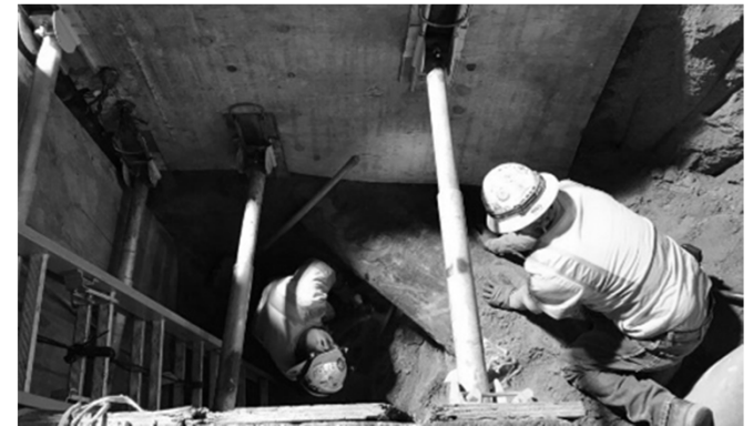
Excavation of 20" waterline on Central Avenue
