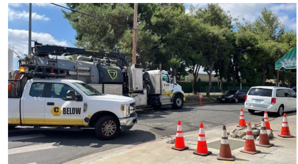
Sidewalk Panel Restoration on Bessemer St
