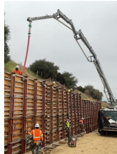
Pouring concrete at Retaining Wall 2461
