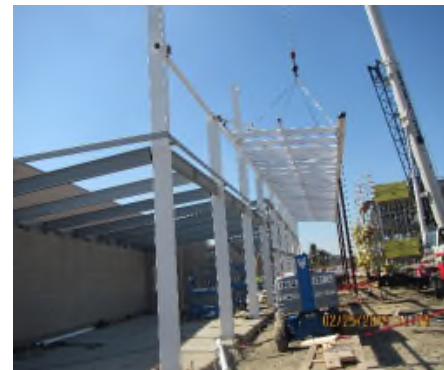
Structural Steel Installation for Mobility Hub
