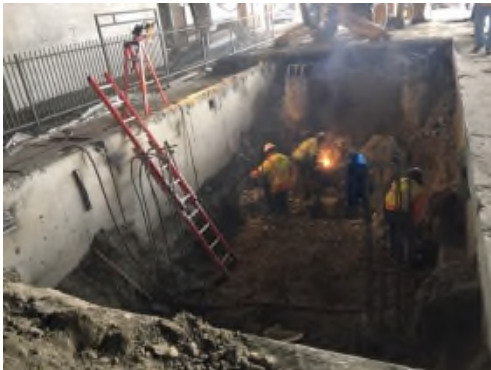
Demolition of Rail Platform
