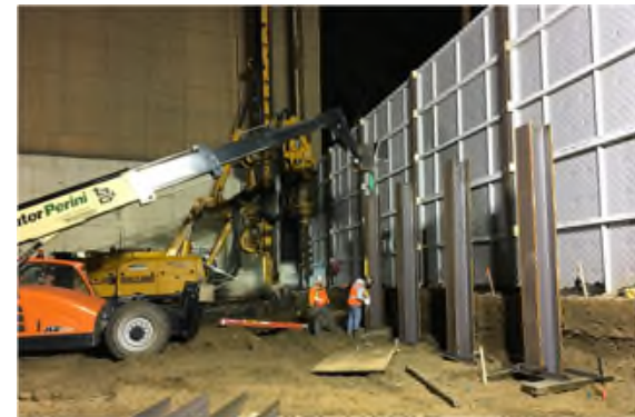
Muck Bin Pile Installation
