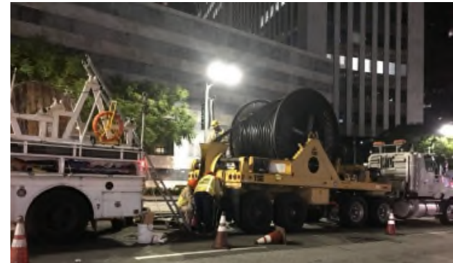
LADWP Cable Pulling
