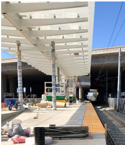
Blue Line Platform Work
