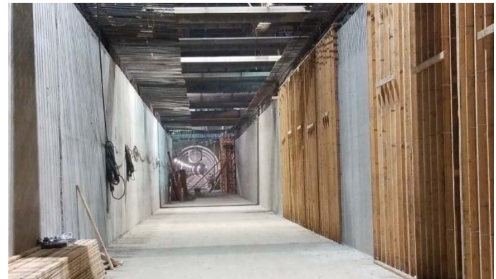
Left track tunnel at Flower St
