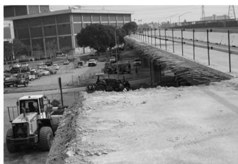
Edge of Deck Removal
