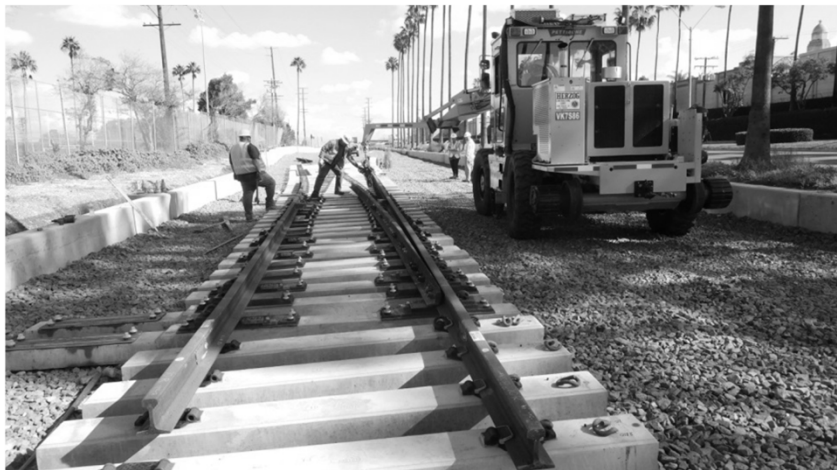
Special trackwork has commenced in Inglewood right-of-way HDPE liner installation at north portal near Leimert Park
