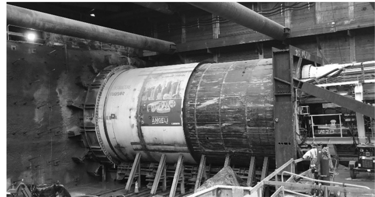
TBM mining underway
