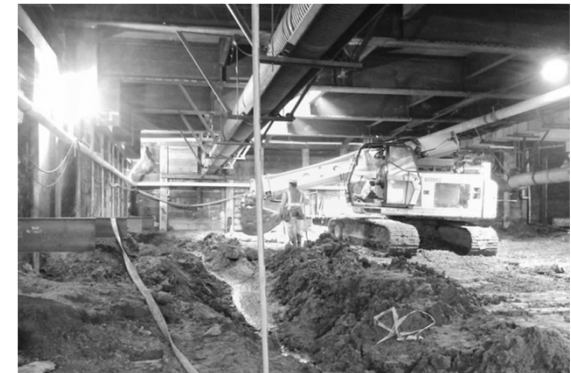
Excavation at Wilshire/La Brea Station
