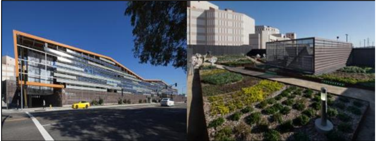
Figure 11: Division 13 - Bus operations and maintenance facility
