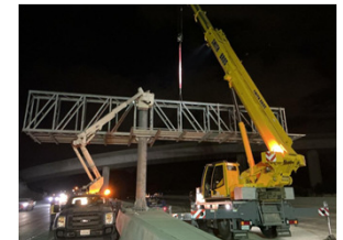
Sign Structure Truss Installation
