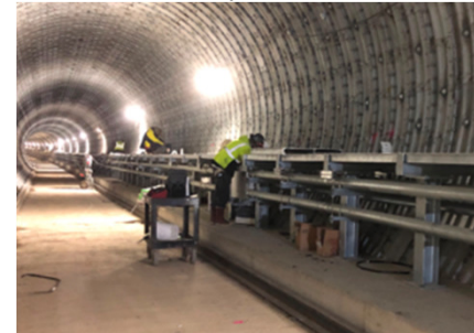
Tunnels: Steel Walkway Construction BL Tunnel
