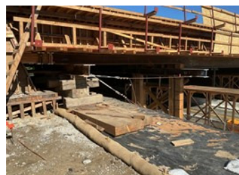
105EB stanford bridge falsework
