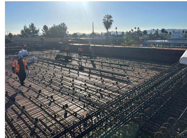
Rebar Installation at Van Nuys Bridge
