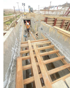
Drain System 406 Formwork Install
