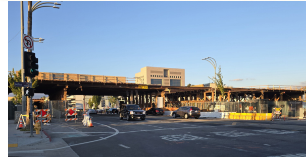
Falsework for Van Nuys Bridge
