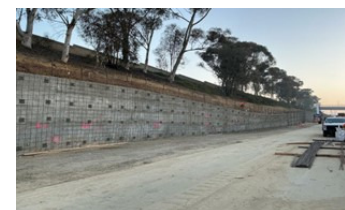
105WB RW 270 Soil Nail Wall Exterior
