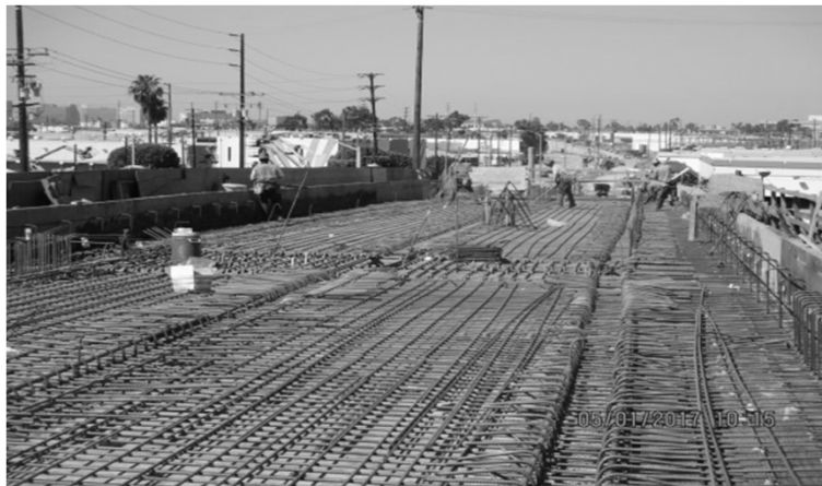
Preparing for a deck pour on the I-405 bridge structure.
