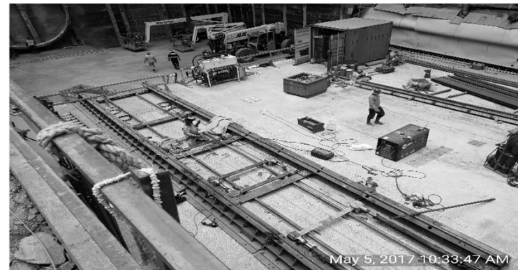
Installing/Staging Reception Cradles in 2 nd /Hope Station
