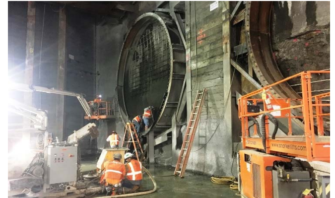
Preparing for TBM Arrival at Wilshire/Western
