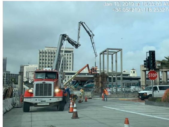
Pouring columns for the elevator structure
