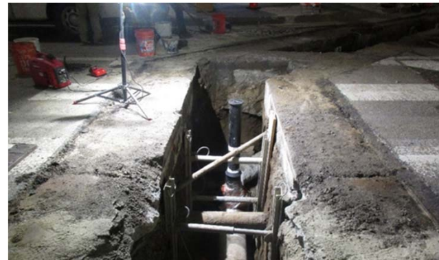
Gate Valve Steel Lateral Utility Installation
