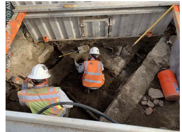
Investigation of the ESA at the west end of the retaining wall
