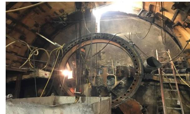
North Tunnel TBM Cutterhead Removal
