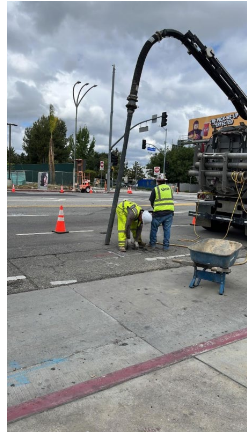
Potholing at Van Nuys Blvd
