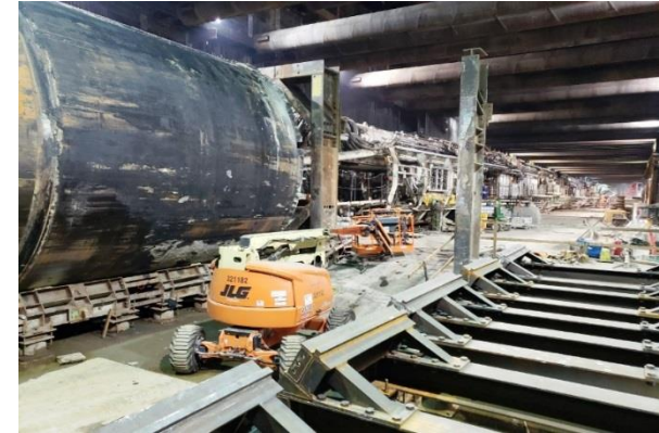
Purple TBM at Wilshire/Fairfax Station
