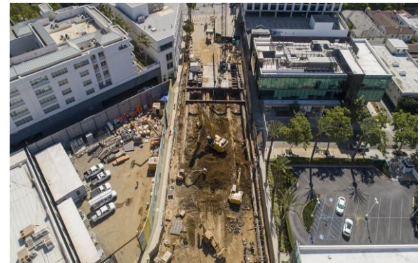
Street Decking Installation on Wilshire Boulevard
