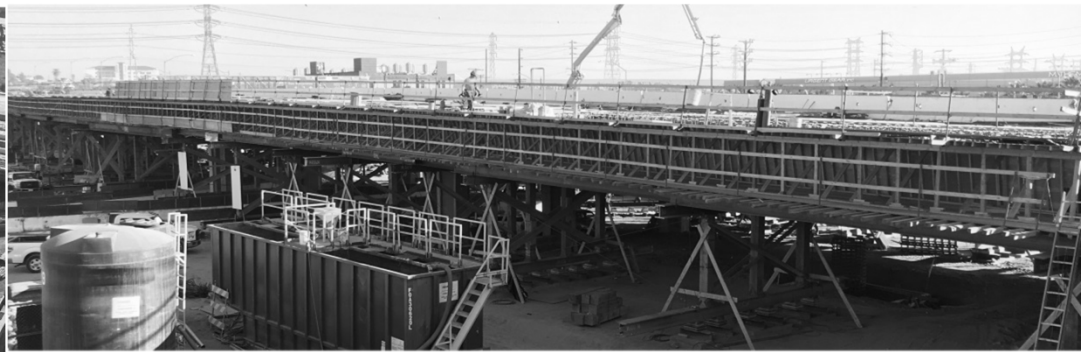
Falsework – Left Side
