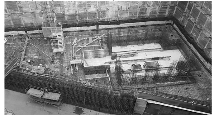
Invert pour and rebar installation at Grand Av Arts/Bunker Hill Station
