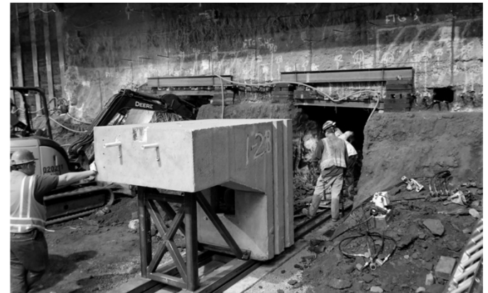
Underpinning activities underway at Historic Broadway Station
