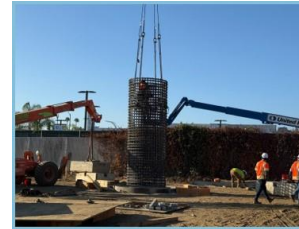
Setting Column Cage at Van Nuys Bent 25
