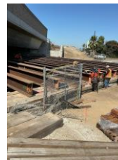
105WB-Dominguez Channel - Setting falsework beams
