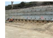
105WB-RW270 - Installing weepholes with geo-composite drain strips with meshing on row 4
