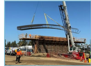
Setting Reinforcing Steel at Van Nuys Abutment 5
