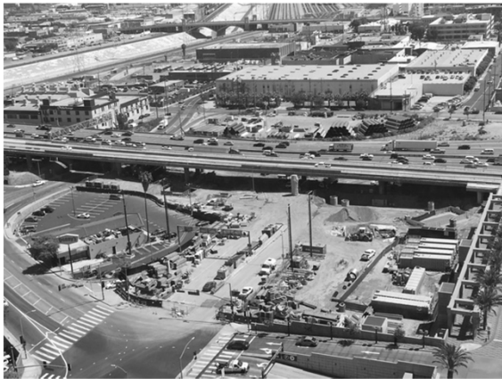
Aerial view of site
