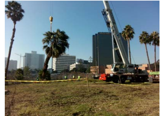
Tree Removal at VA Site
