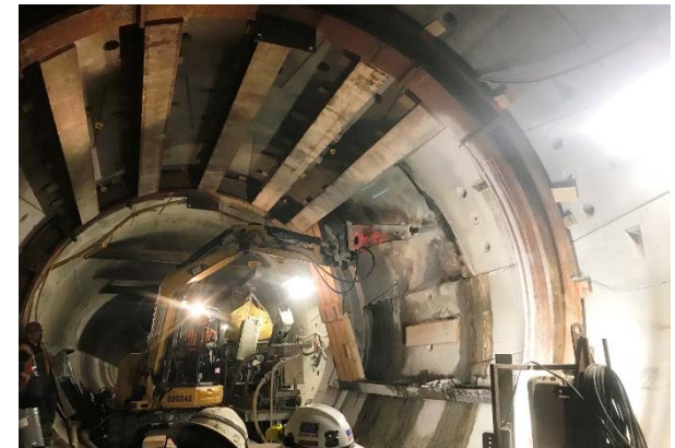
Excavation at Cross Passage 10
