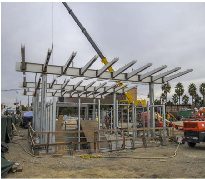
EXPO/CRENSHAW STATION – Canopy over main station entrance
