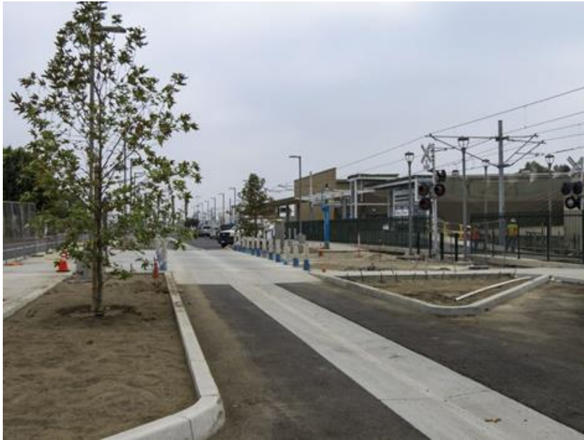
Fairview Heights Station - parking, landscaping, and pedestrian crossing
