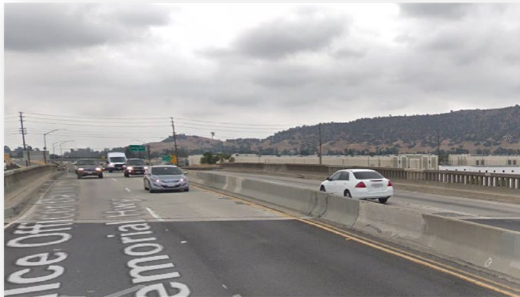
BEFORE Rail Bridge Construction
