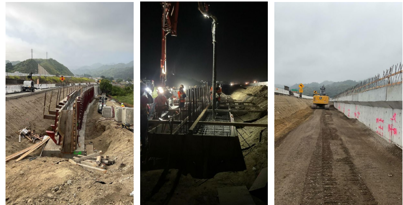
On-going work at Retaining Wall 2577
