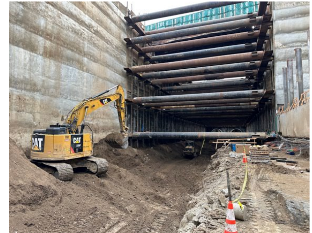
Westwood/VA Hospital Station: Excavation in Station Box
