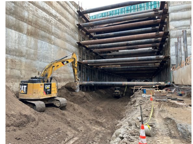
Westwood/VA Hospital Station: Excavation in Station Box
