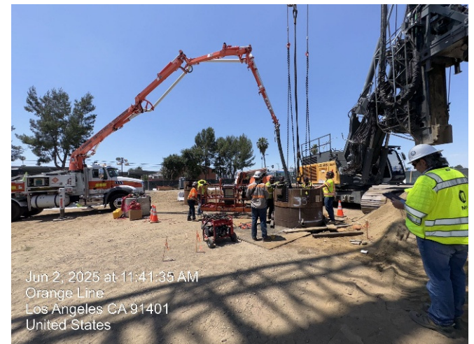
CIDH Foundation Installation at Van Nuys
