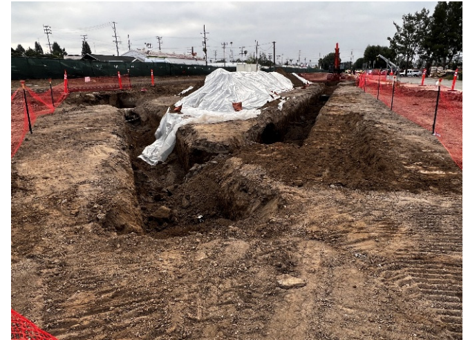
Storm Drain Removal at Van Nuys
