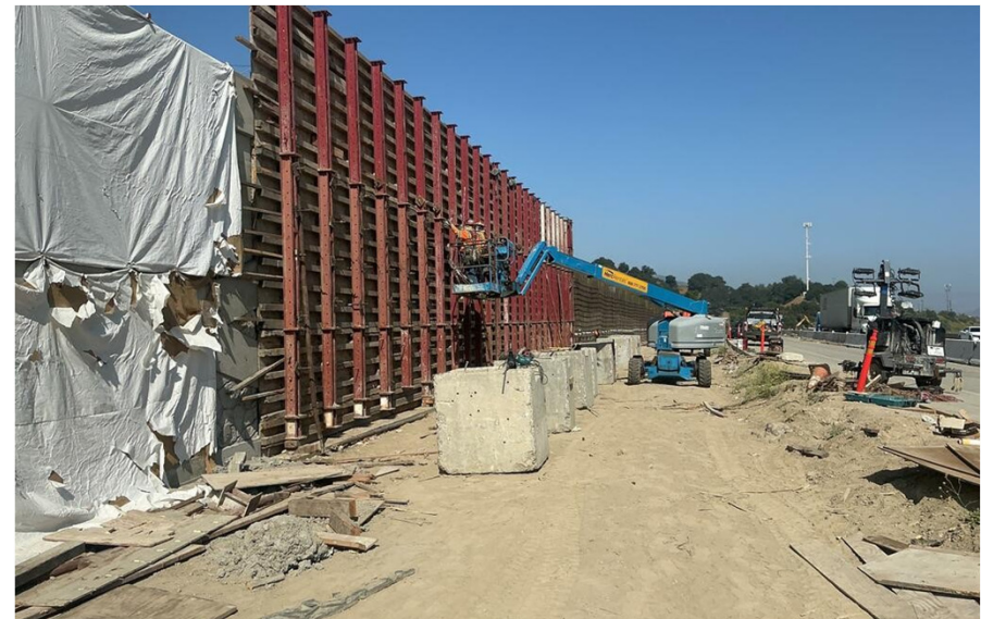
Retaining Wall 2449 Formwork Installation
