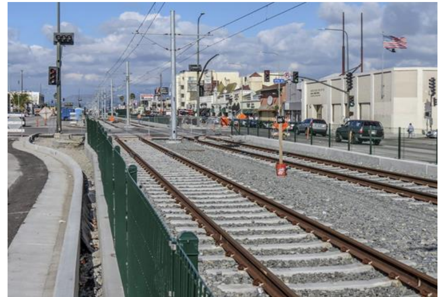
Trackwork and overhead catenary system – Crenshaw & 57 th
