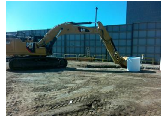
Excavation of TTES Guide Wall Trench
