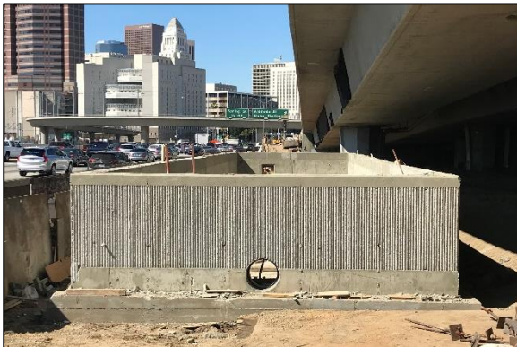
Austin Vault completed
