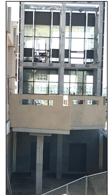
Elevator glass enclosure completed
