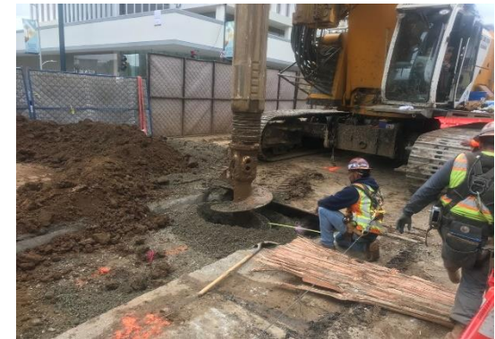
Pile Installation at Wilshire/Rodeo Station
