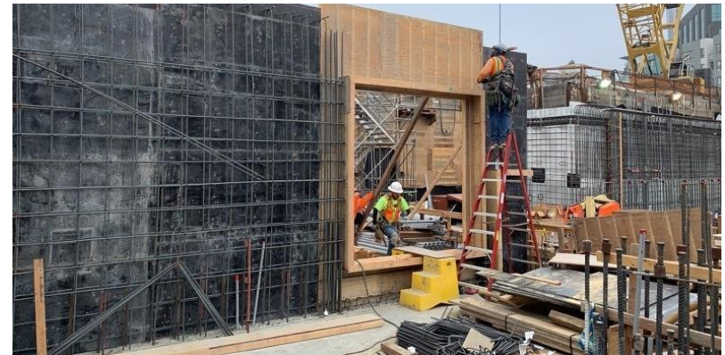
Fan Room interior wall construction at future Little Tokyo/Arts District Station
