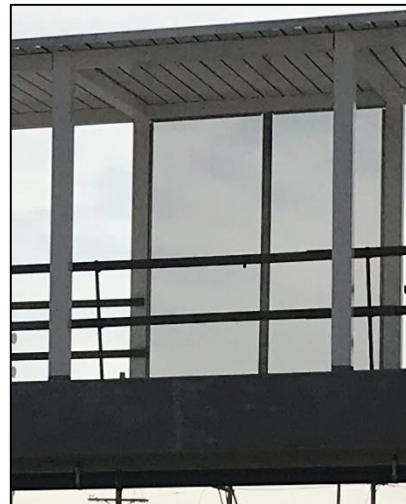
Interior panels initiated
