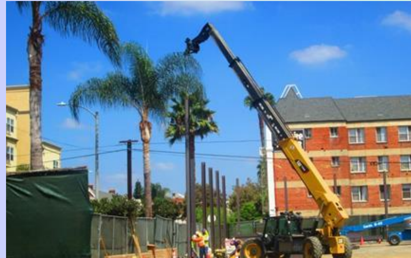
Soundwall Construction at North Wilshire/La Brea
