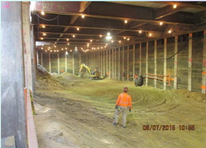
LEIMERT PARK STATION – Excavation and lagging
