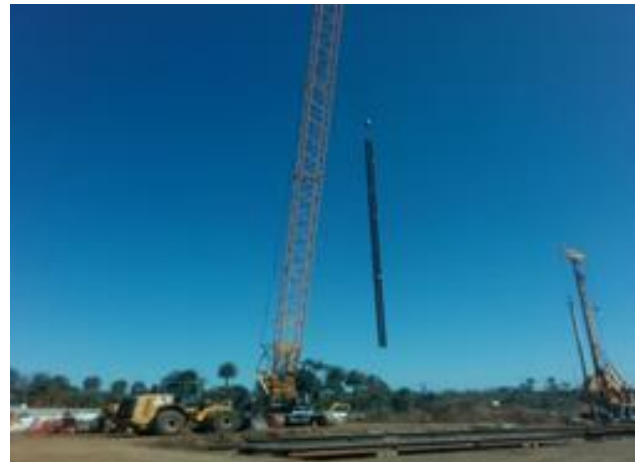
Support of Excavation (SOE) Pile Installation at VA
