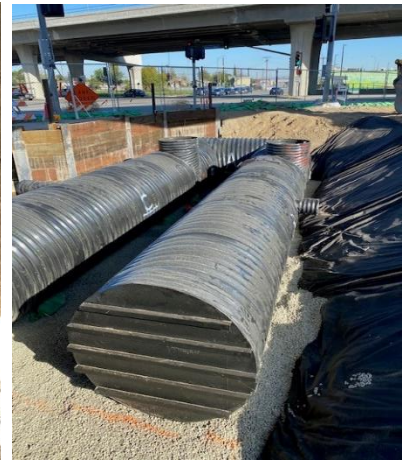
Installed cistern for North GSRD
