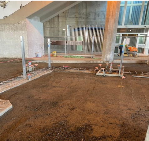
Completed underground utility work @ C Line west
