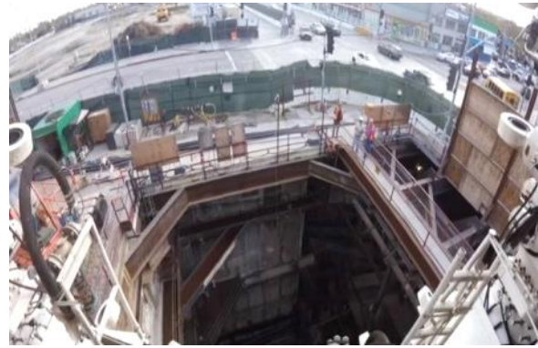
Example of a Construction Staging Site
