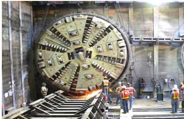
Tunnel Boring Machine
