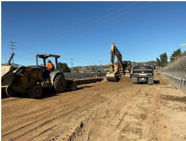
Calgrove Off-Ramp Gore Area Concrete Preparation
