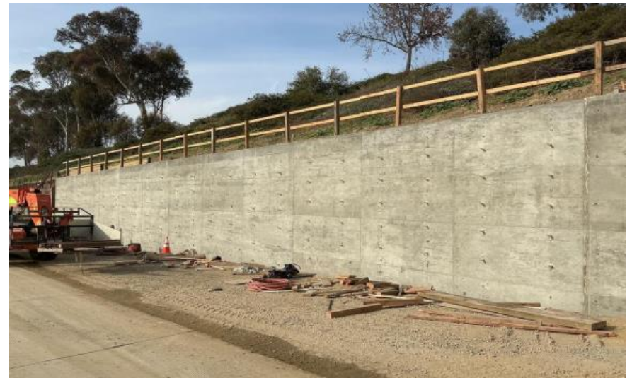
Stripping of forms from retaining wall
