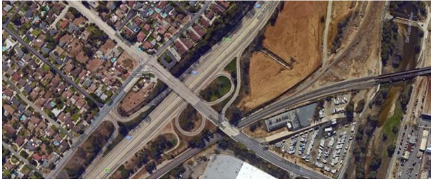
Aerial View of Existing Beverly Blvd.
