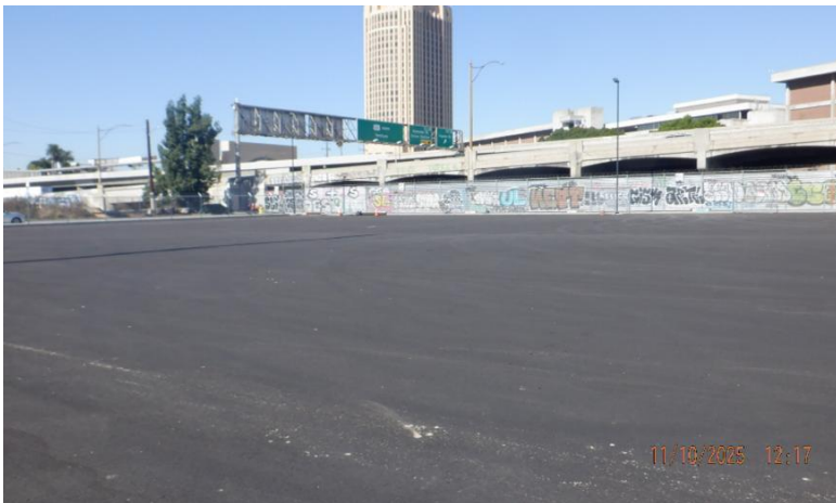
Building demolition & site paving complete (December 2025)
