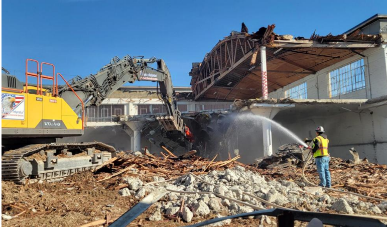
Life Storage building demolition (March 2025)
