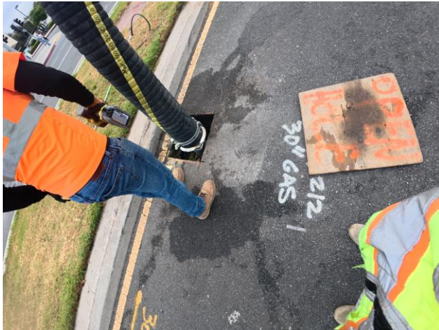
Potholing Early Works Package in Glendale
