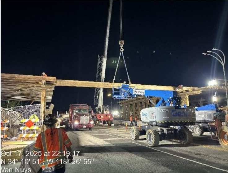
Setting Bents and Welding Stringers at Van Nuys
