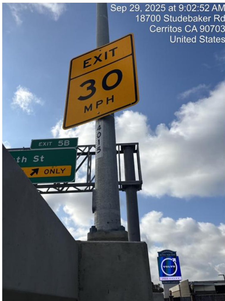
Final South Street lighting and signage
