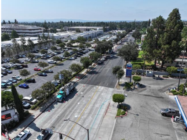
Potholing Early Works Package in Pasadena
