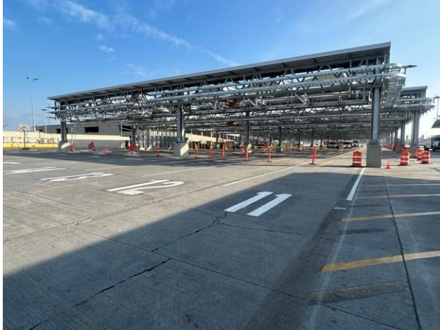
Division 9 Charging Station
