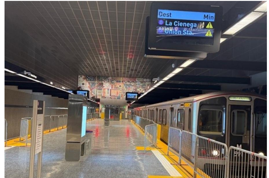
Test Train at Wilshire/La Cienega Station Platform
