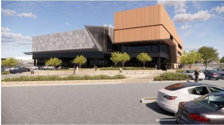
Building Exterior - West View
